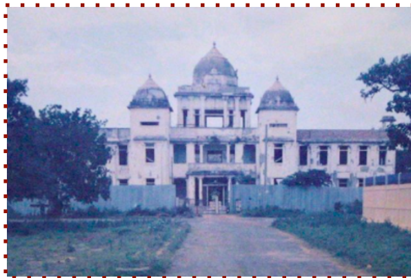
« Jaffna Public Library - « A view after 1981 destruction » - a framed display which hangs in the library today. »
